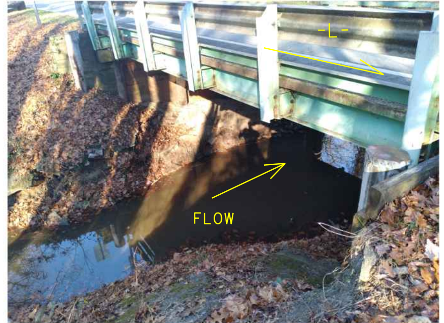
Photo #4: Bridge 198 south side looking west (downstation)
