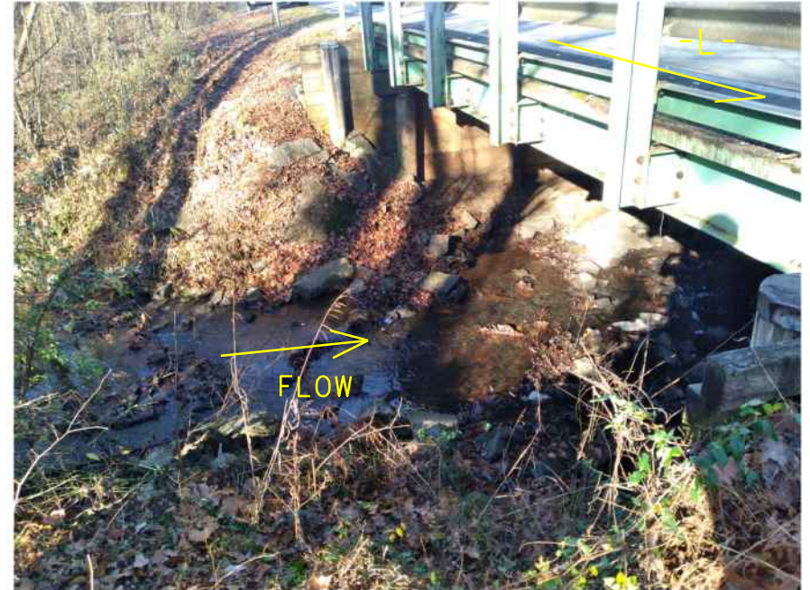
Photo #2: Bridge 199 south side looking west (downstation)
