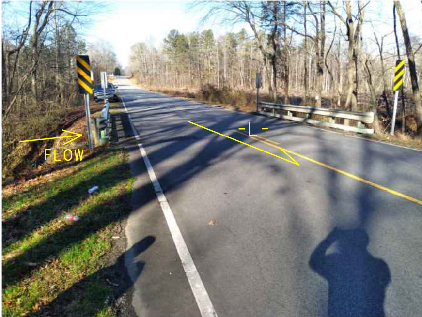
Photo #1: Bridge 199 End Bent 2 looking west (downstation) towards End Bent 1
