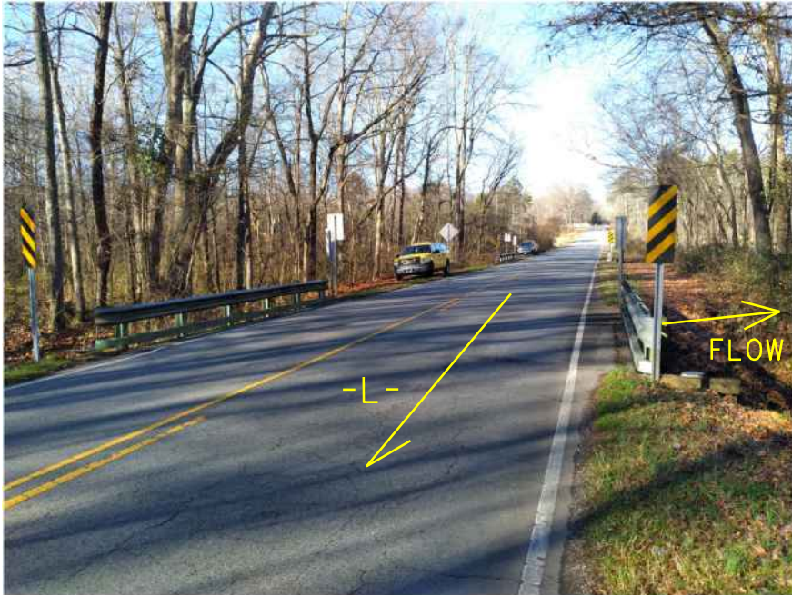
Photo #3: Bridge 198 End Bent 2 looking west (downstation) towards End Bent 1
